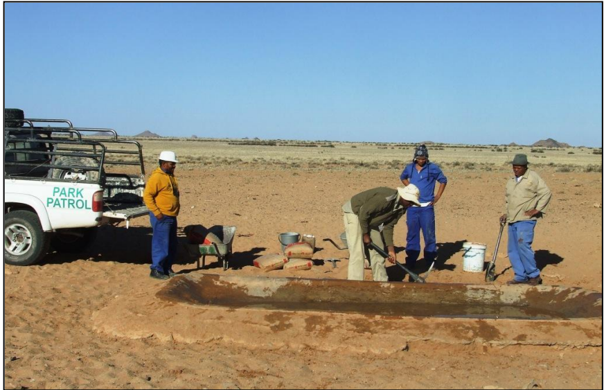
Repairing Dassiepoort waterhole
