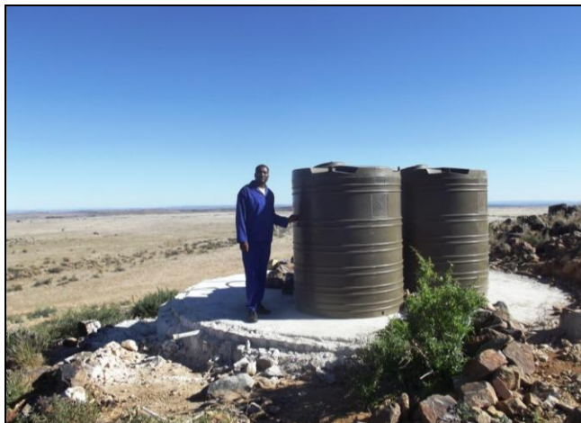
Ranger Epafra Akwenye by the completed tanks
