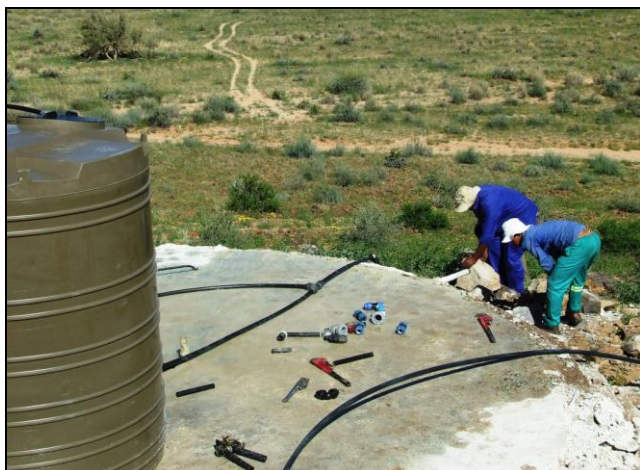
Fitting the new water tanks at Dassiepoort
