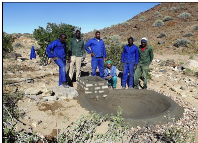
Waterhole construction at Brakwater
