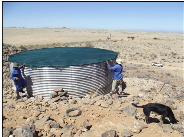
Fitting shade cloth over Dassiepoort reservoir
