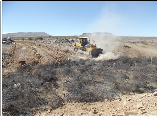
Bulldozer filling the hole with house rubble and soil
