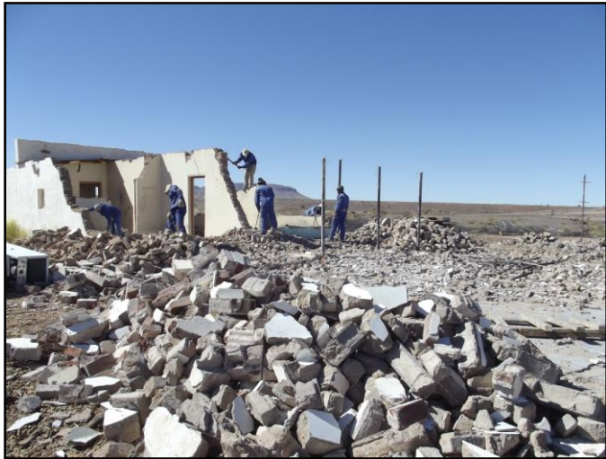
Demolition of Geluk house
