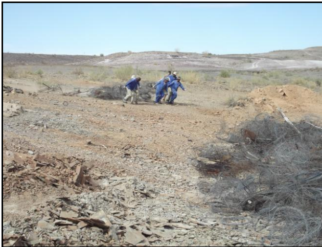
Pulling wire into the hole made by the bulldozer
